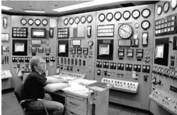
Boiler Operator Jeff Craigie sits in the Boiler Room and monitors flows, temperatures and pressures of the boilers and feed-water system. Photo by Peter Schmitt
